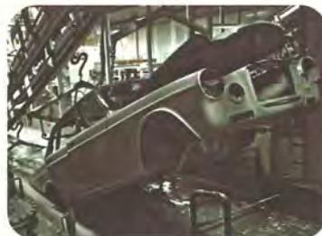
The body is rustproofed inside and out by completely submerging it in this special primer. An electrolytic process causes the steel to attract the paint in a thick, even layer.
