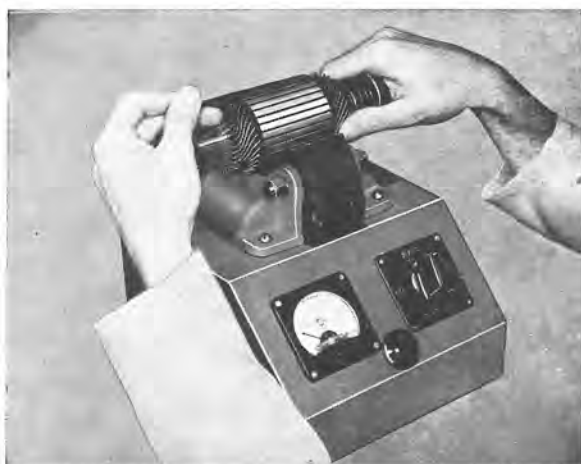
Fig. 3-40. Testing armature
