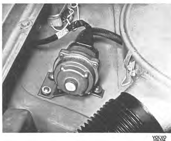
Fig. 2-115. Pressure sensor installed
