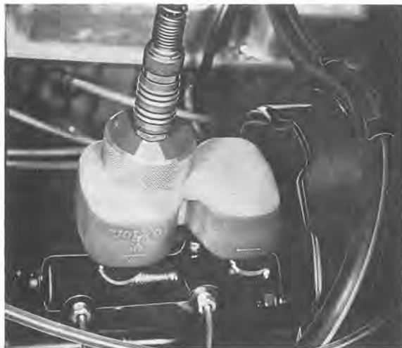
Fig. 5-61. Connecting bleeder unit
